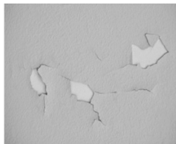
Enamel and latex based paints typically flake or chip in strips and peel away.
